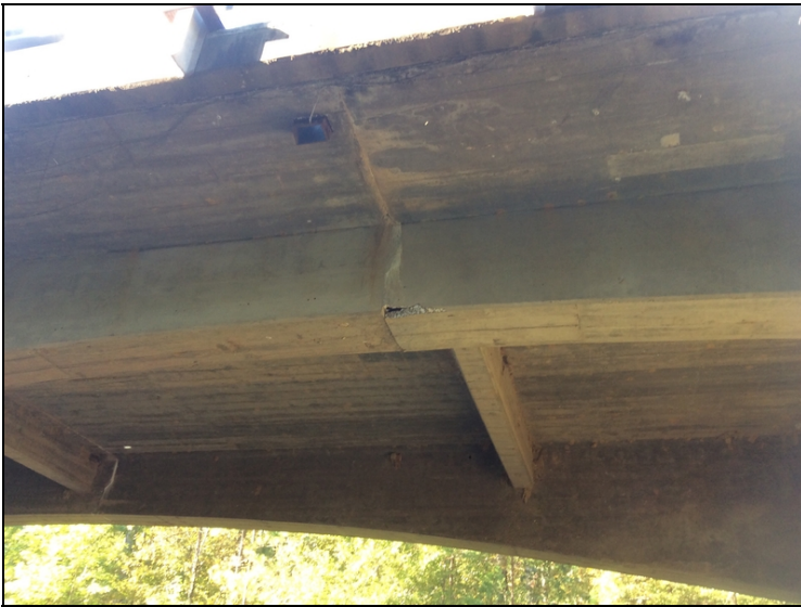
Span 2, girder 2. Exposed rebar at mid span.
