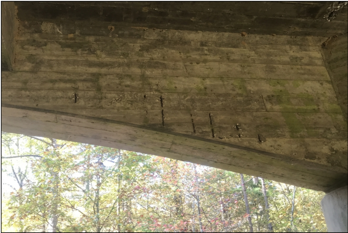
Span 1 girder 1 right side has spalls with exposed rebar.
