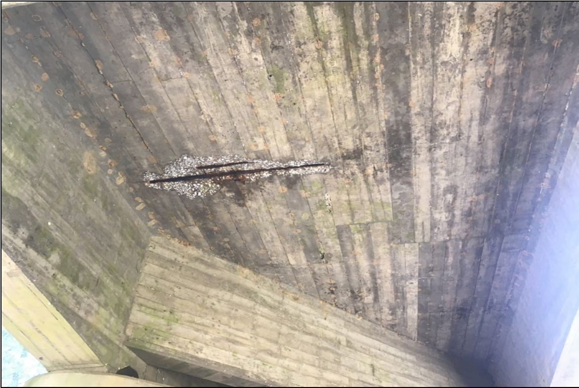
Span 2 soffit has spall with exposed rebar.
