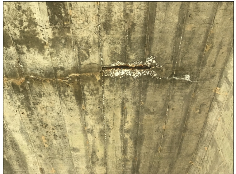
Span 3 soffit has spall with exposed rebar.
