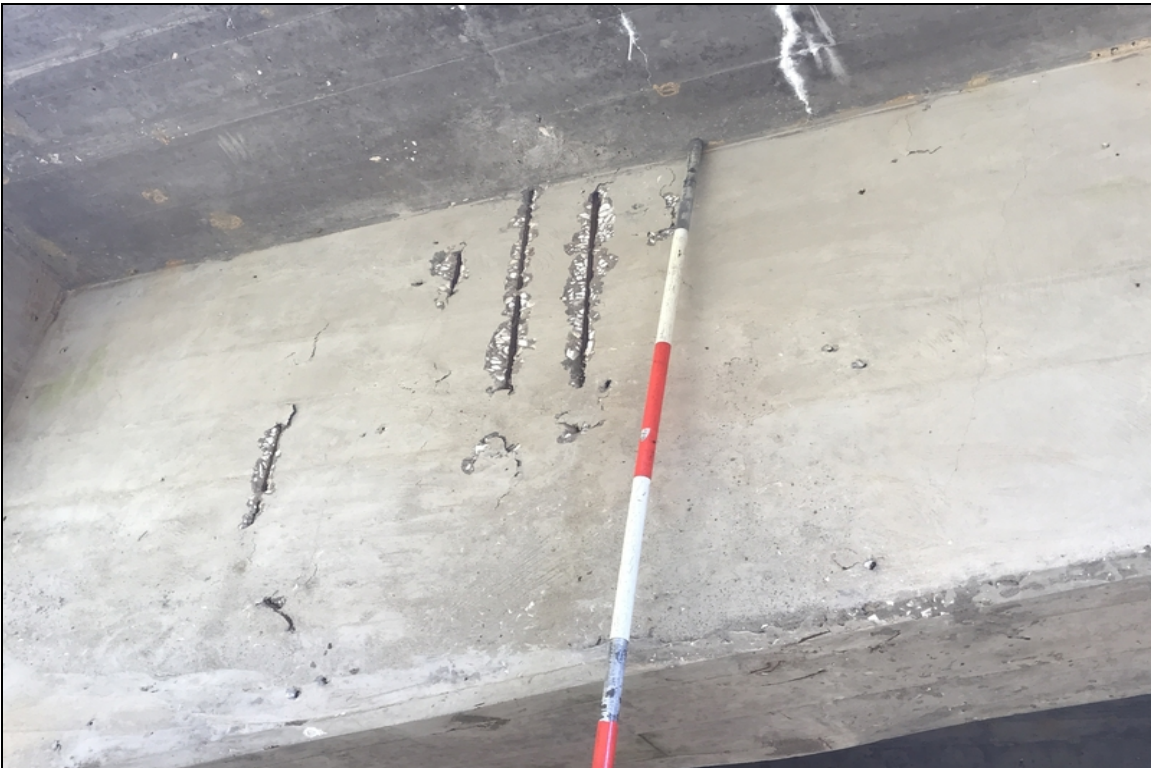
Span 2 girder 1 at bent 3 left side has spalls with exposed rebar.
