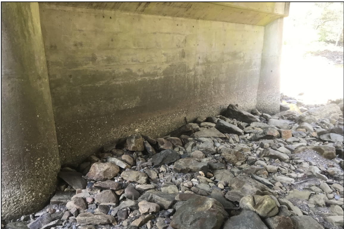
Bent 2 pier wall has abrasion at ground level.
