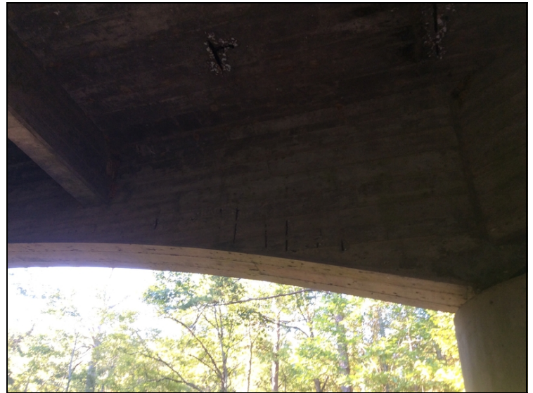
Span 1, girder 1, inside face. Spalls with exposed rebar.
