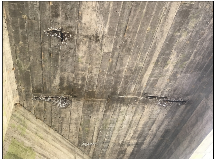
Span 1 soffit has spalls with exposed rebar.
