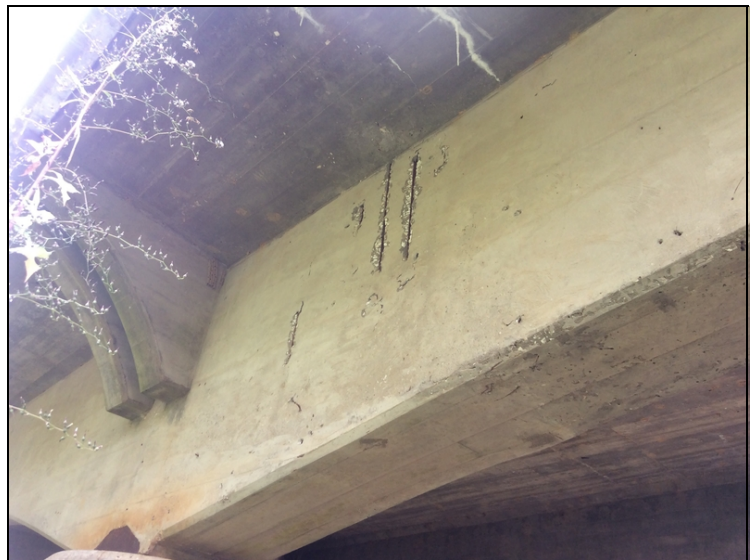
Span 2 Girder 1 left side spalls with exposed rebar.
