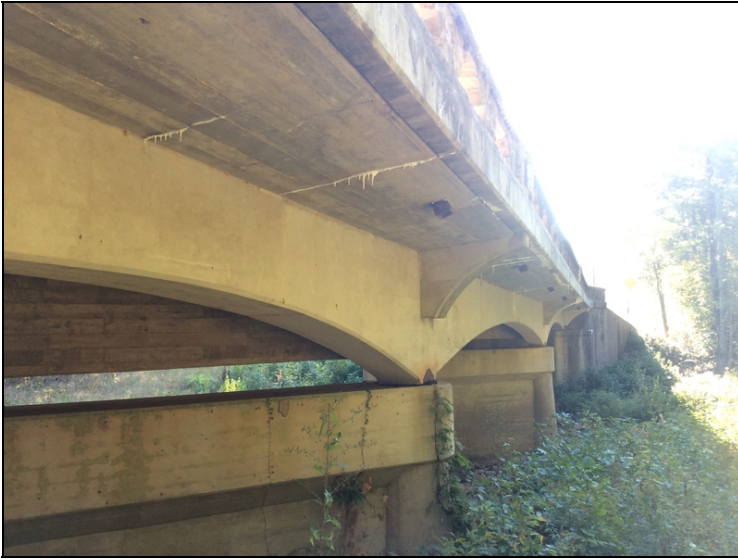
Left side looking back. Efflorescence on all three spans.
