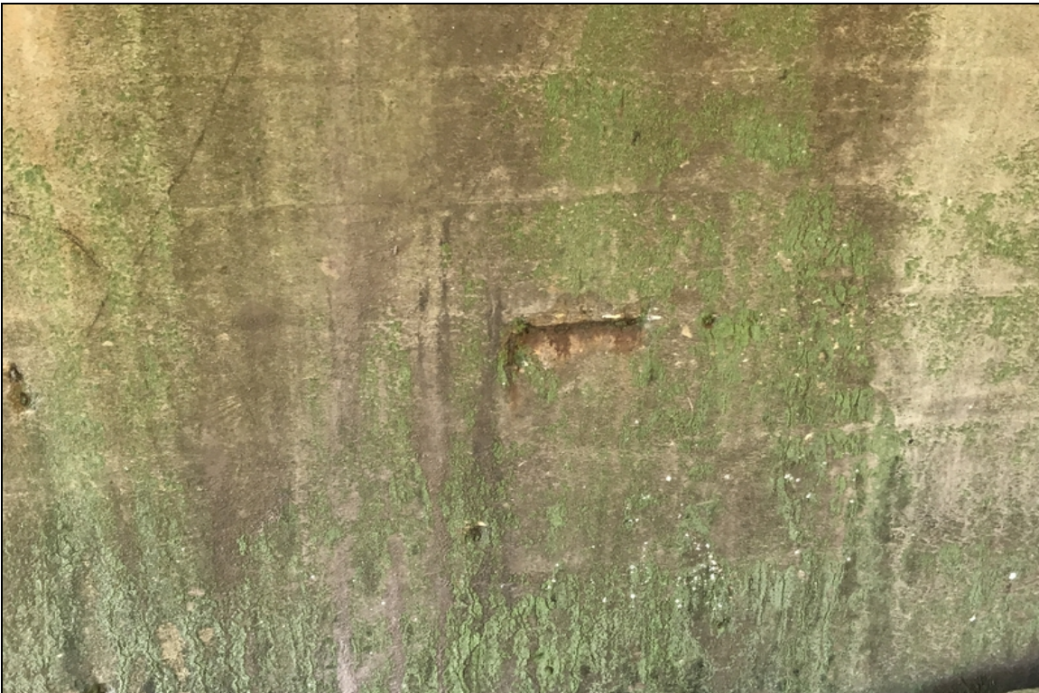
Bent 4 abutment has spall with exposed rebar.
