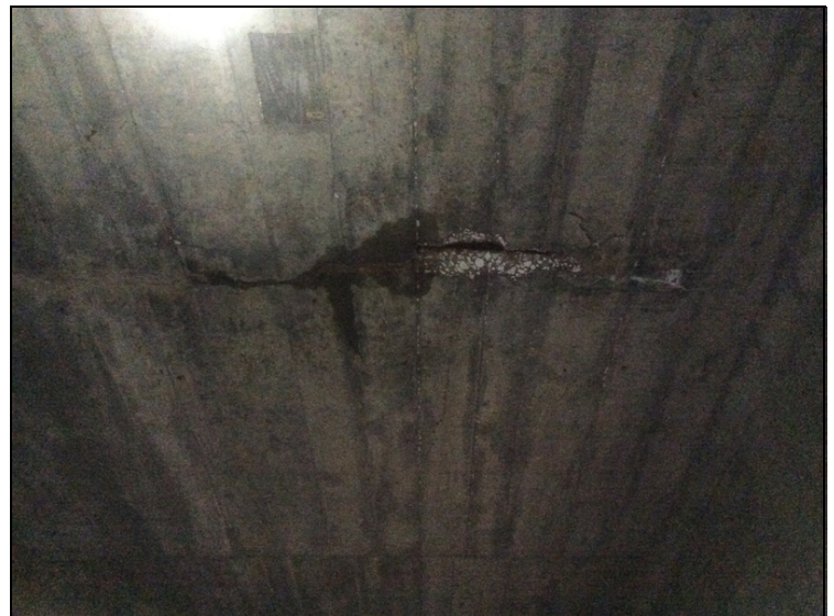
Span 3, spall with exposed rebar in the soffit.
