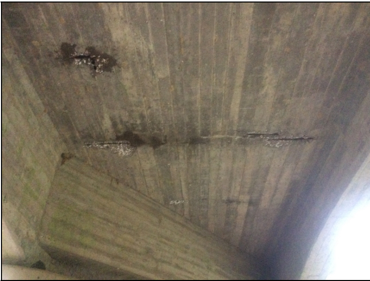
Span 1, spalls with exposed rebar.
