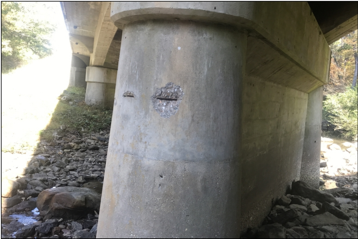
Bent 2 column 1 has spall with exposed rebar.
