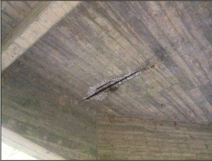
Span 2, large spall with exposed rebar.
