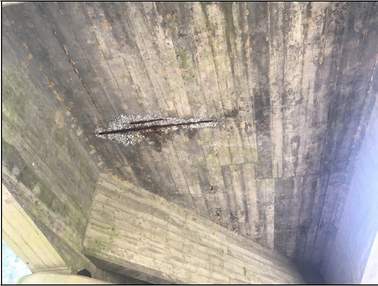
Span 2 soffit has spall with exposed rebar.
