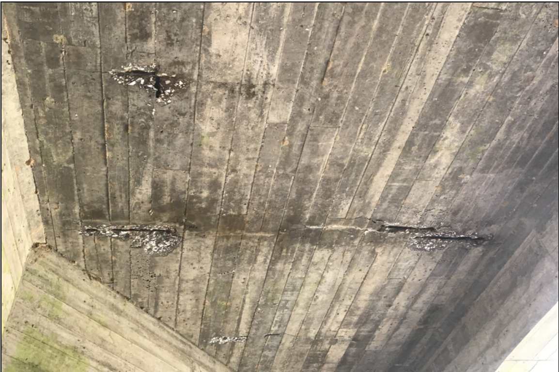
Span 1 soffit has spalls with exposed rebar.
