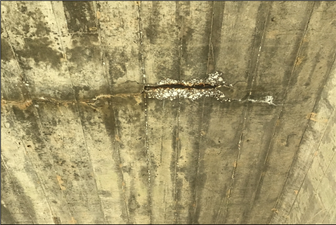
Span 3 soffit has spall with exposed rebar.
