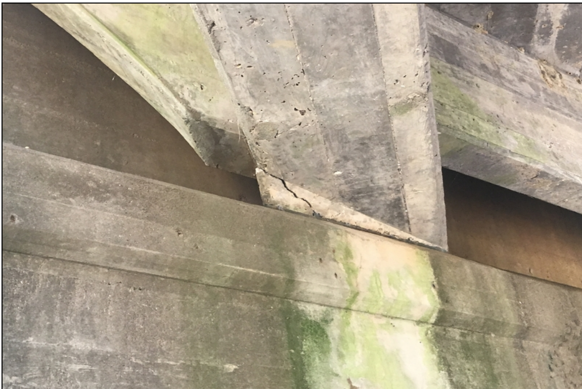
Girder 2 at bent 1 has delam above bearing
