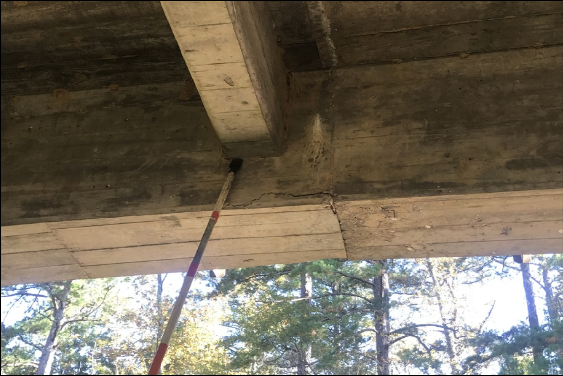
Span 2 girder 2 has delam at mid span.
